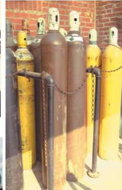
Figure 25-37 Cylinders present additional risks to responders because not only can the contents be hazardous, but if the cylinder is involved in a fire it may explode.
